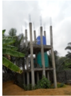
Water tank – work in progress
