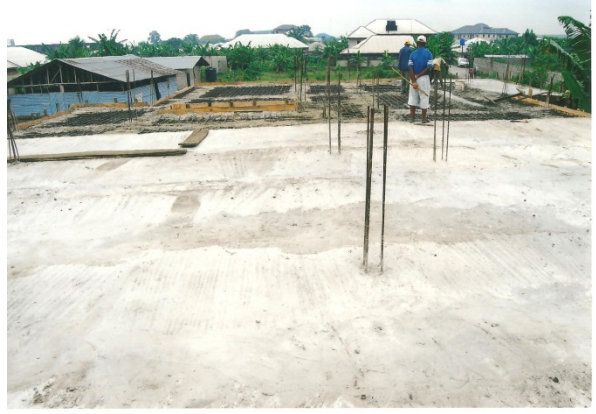
Putting down the iron rods for strength The surrounding area is now being developed
